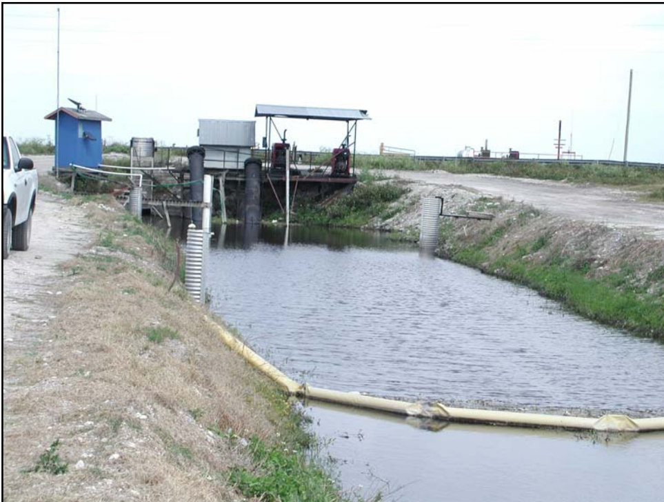
Figure 1.2. Good cleaning program to keep weed away from the pump station
